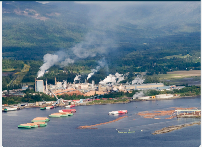
An aerial view of Crofton Mill, a pulp and paper mill located in the Vancouver Island town of Crofton, British Columbia.
