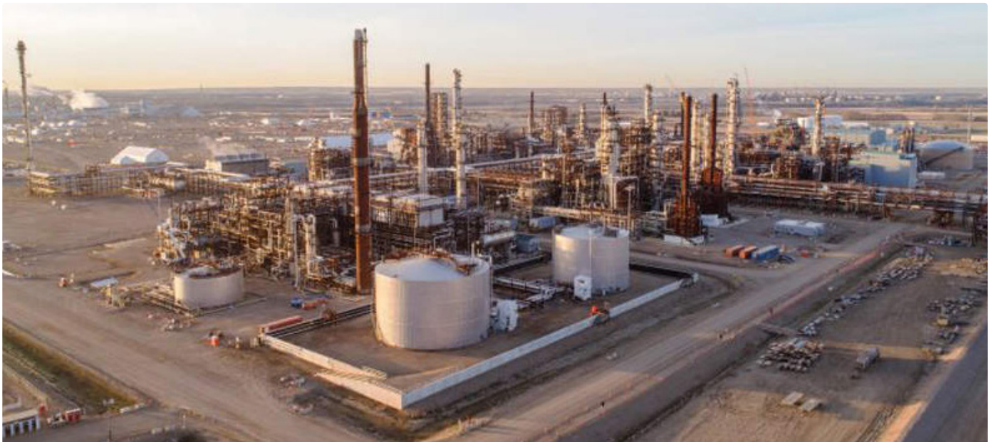
The Alberta Carbon Trunk Line will gather CO 2 from industrial emitters in Western Canada and convey it to reservoirs across Central and Southern Alberta. CO 2 will initially be captured from the Sturgeon refinery complex shown above.
