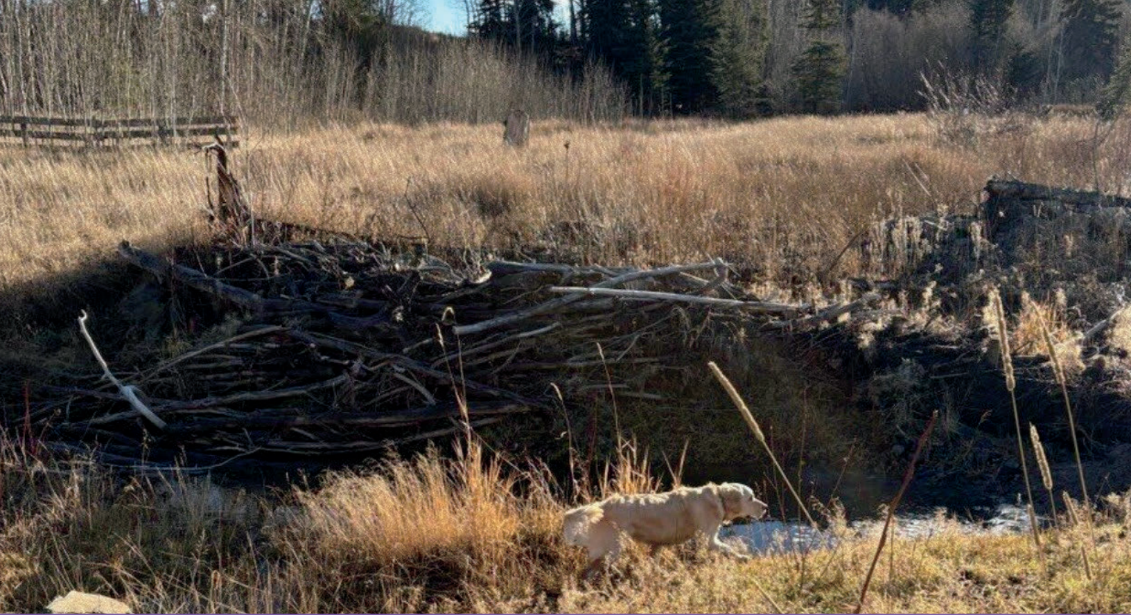
Figure 3. Beaver dam analogue in the field.
