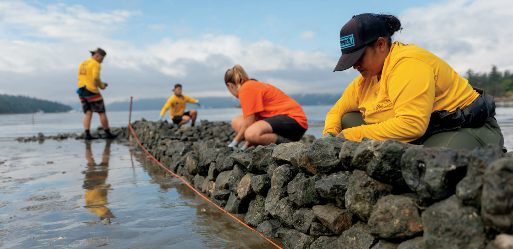
Figure 3. Construction of PFN Sea Garden Wall.
