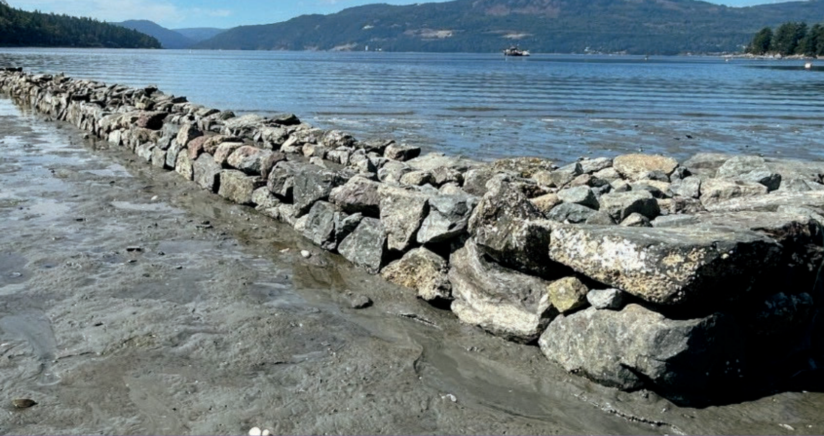
Figure 2. Newly Build PFN Sea Garden Wall.
