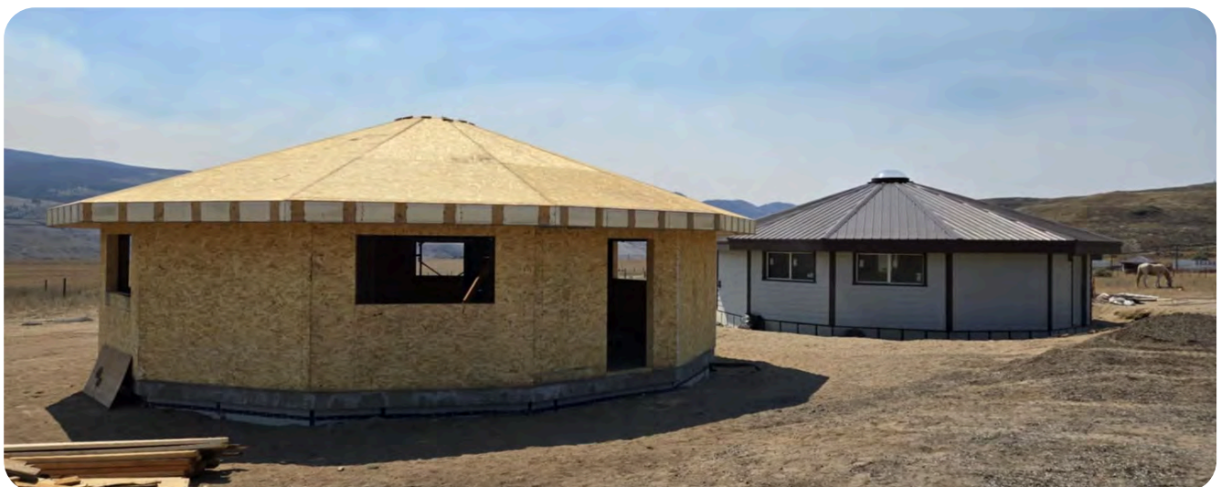
Dodeca-Home under construction. Photo credit: Skeetchestn Dodeca-Homes
