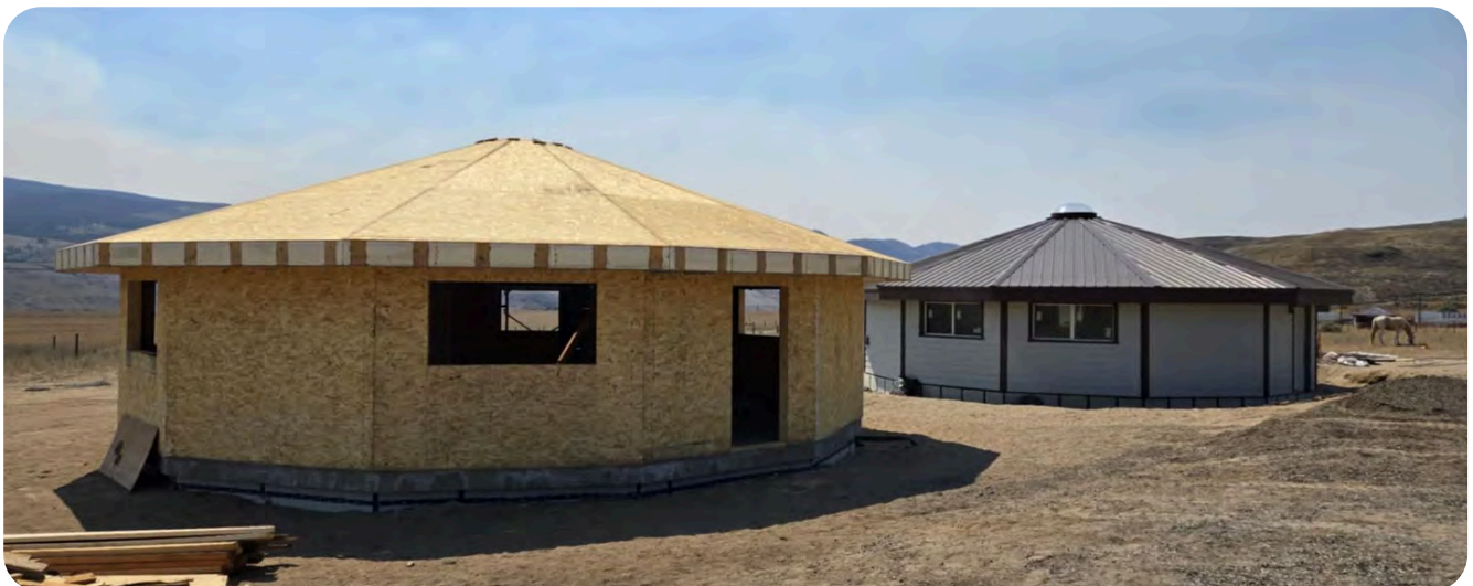
Dodeca-Home under construction. Photo credit: Skeetchestn Dodeca-Homes
