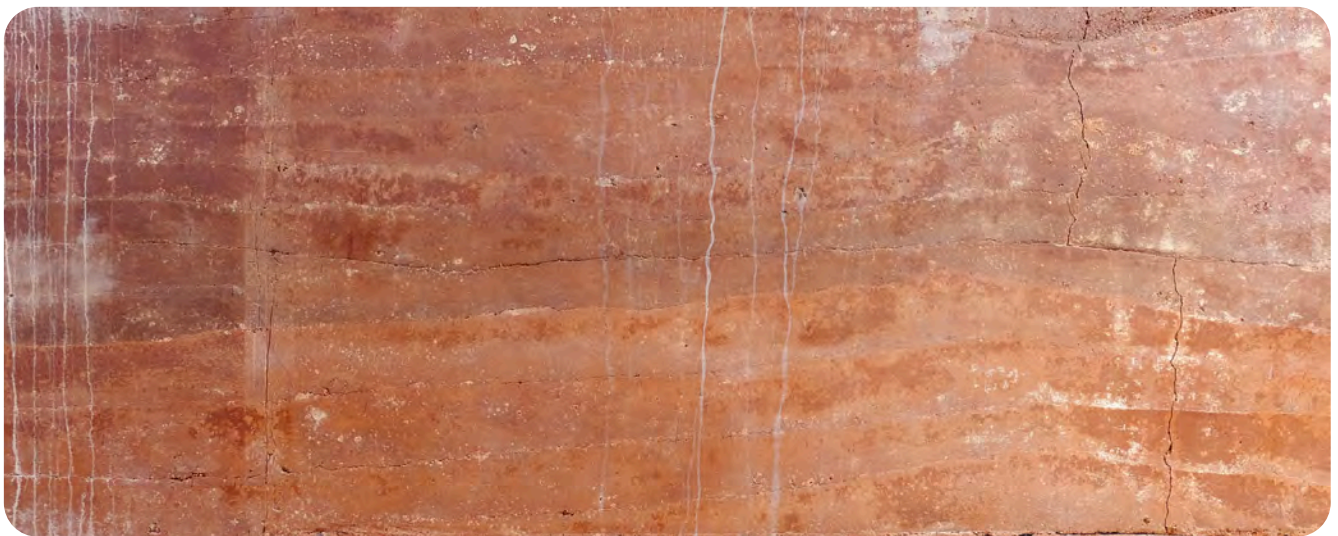
Rammed earth wall
