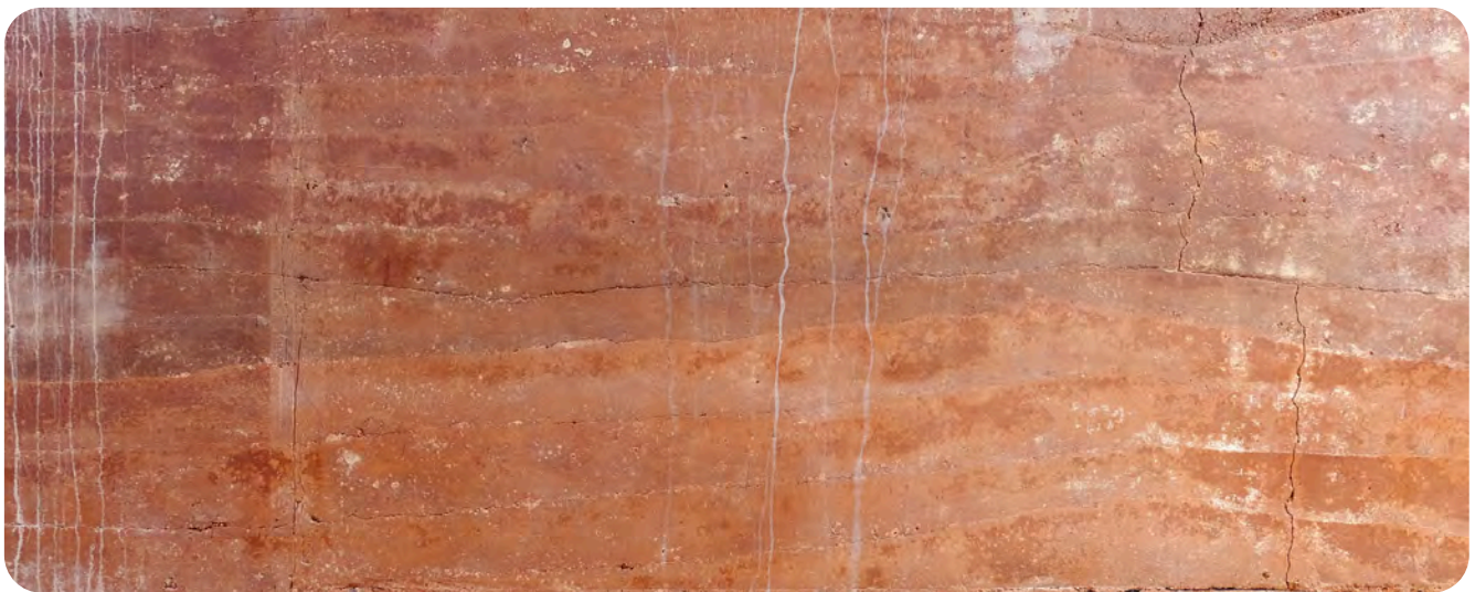
Rammed earth wall
