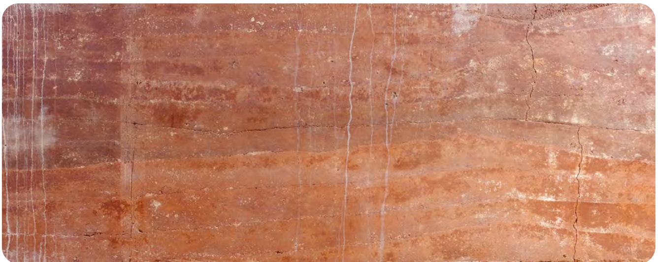
Rammed earth wall
